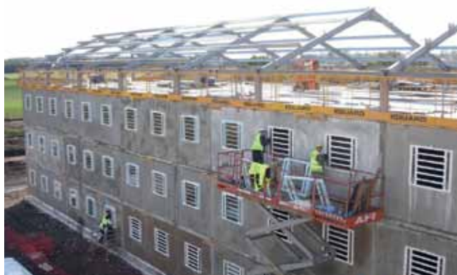
Low Moss under Construction
