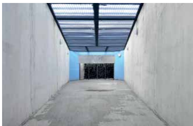
Separation and Reintegration Unit exercise yard HMP Low Moss
